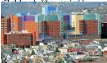
The new campus of Children's Hospital of Pittsburgh of UPMC in the Lawrenceville section of Pittsburgh.
